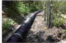
Boulder Creek Diversion Project
