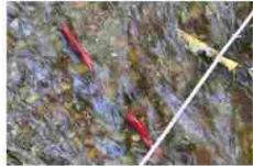
Abel Creek Culvert Rehabilitation Project
